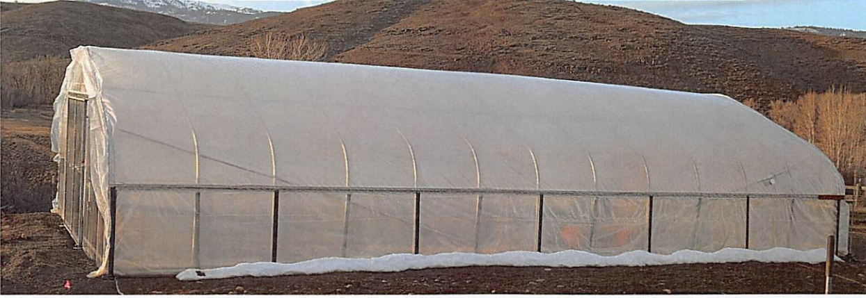
The greenhouse showing the ribs, this structure is 24' wide by 48' long
