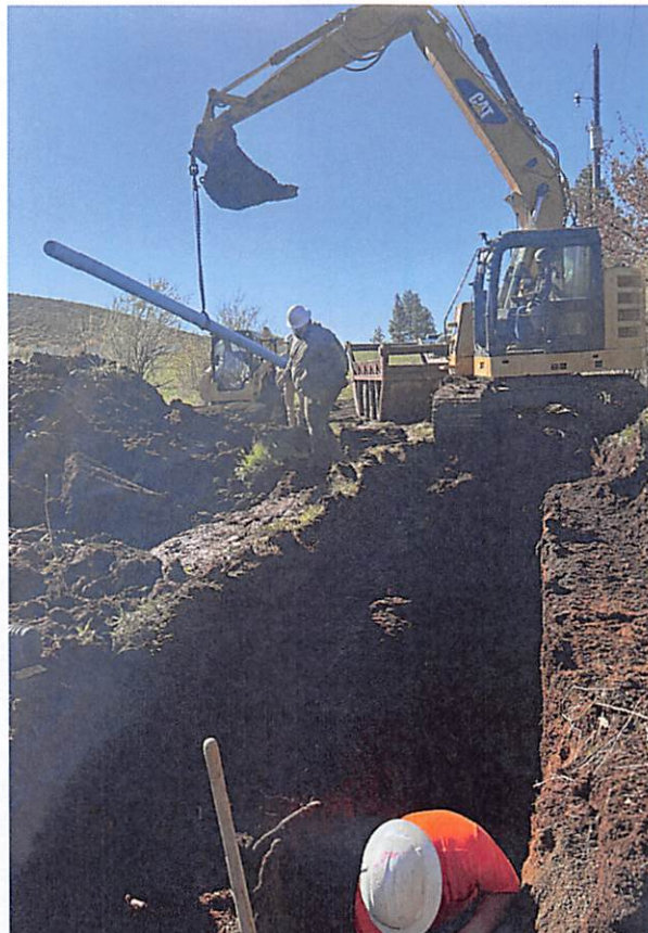
Figure 2: Installation of water main through pasture adjacent to Mountain View Ln
